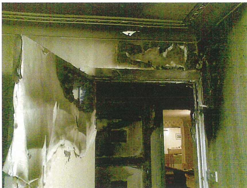
Fire damage in hallway area due to SANAU LPG Cabinet Heater
