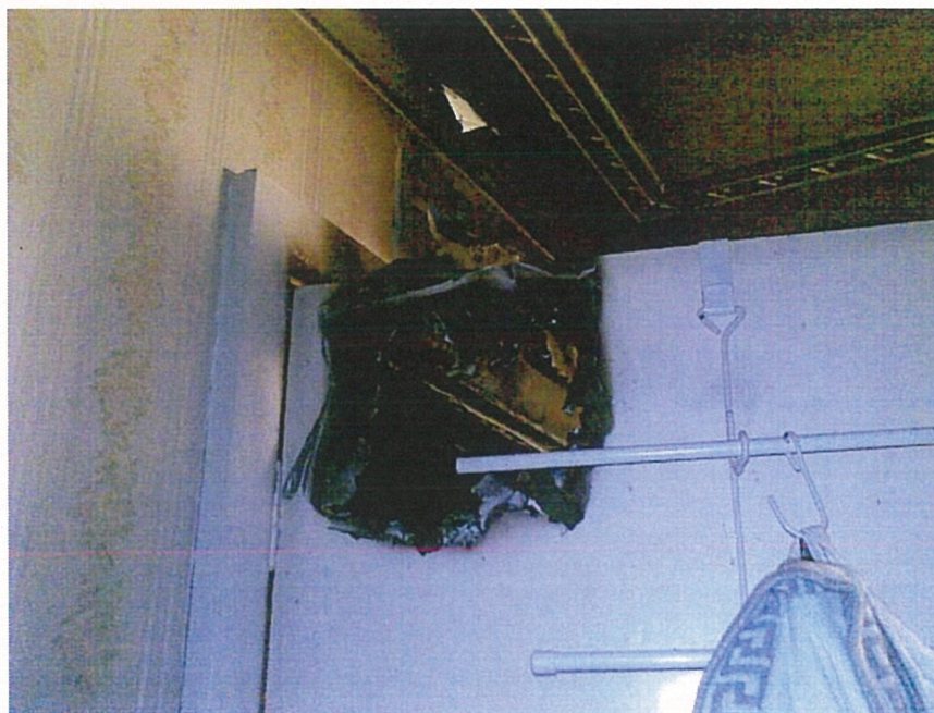
Fire damage in hallway area due to SANAU LPG Cabinet Heater
