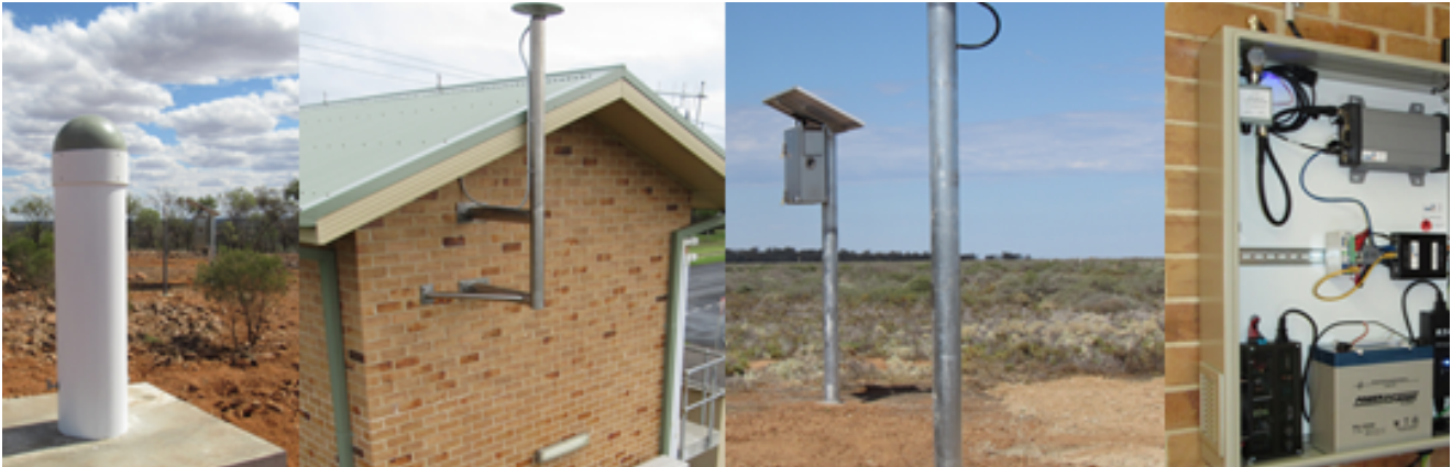
Image typical DFSI Spatial Services CORSnet-NSW installations © DFSI Spatial Services 2018
